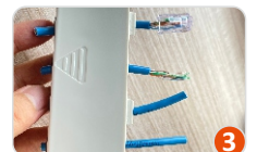
3.Terminate the cable with an RJ45 connector following the T568A or T568B standard.
